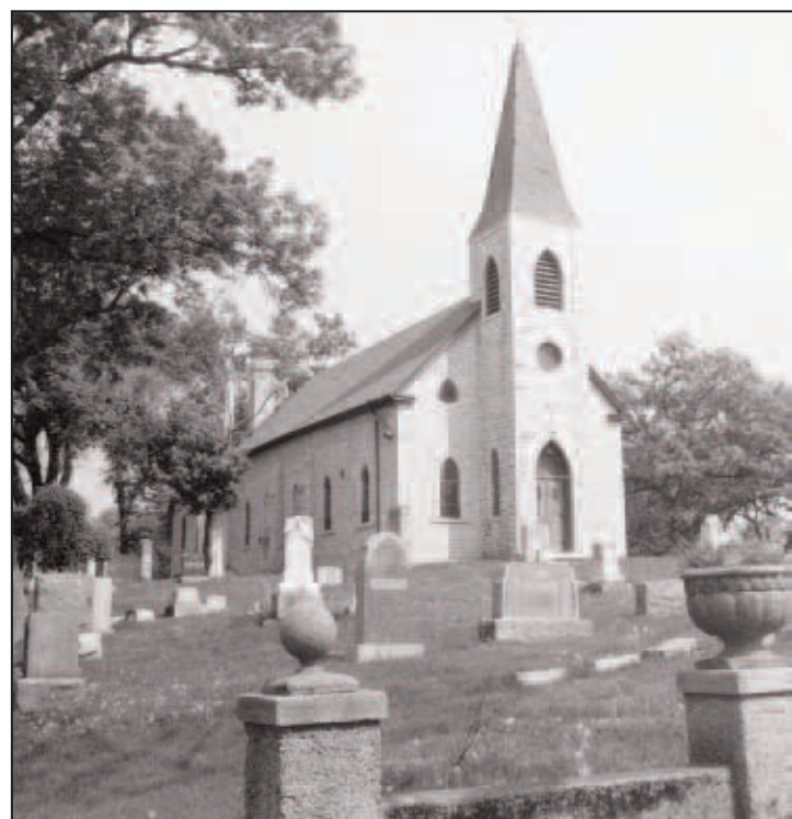
St. James at Sag Bridge Church and Cemetery
